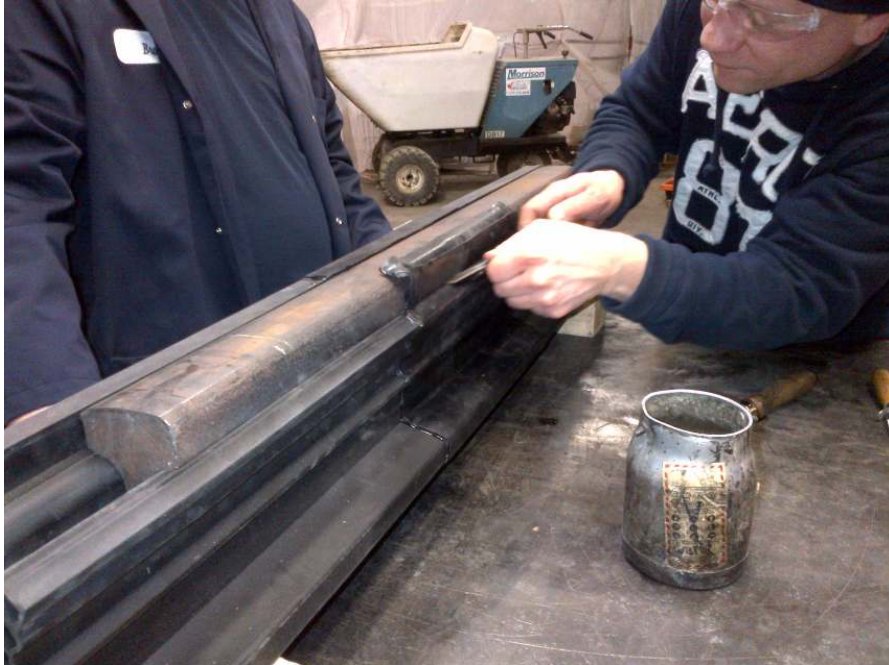
12 - Remove gauge side tape
